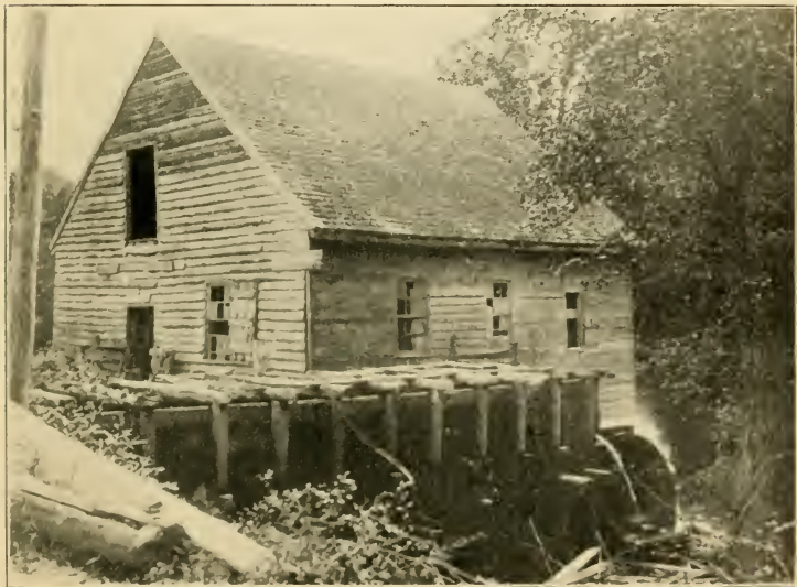
Water-power, "Overshot Wheel," Grist Mill, Richmond Co., Va.
